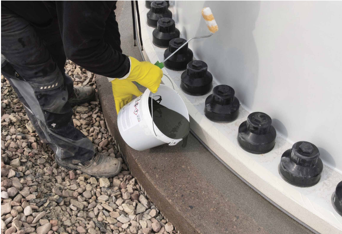
Applying the first layer of KEMPEROL waterproofing.
