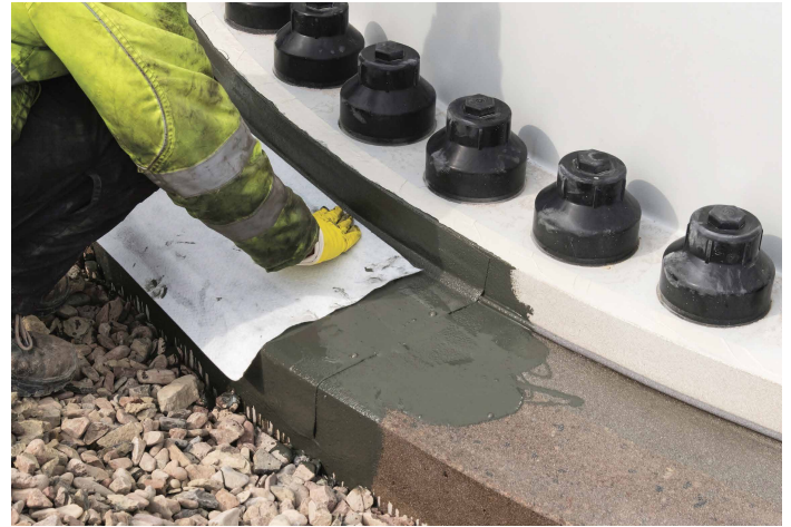
Working the surface fleece into the KEMPEROL layer.
