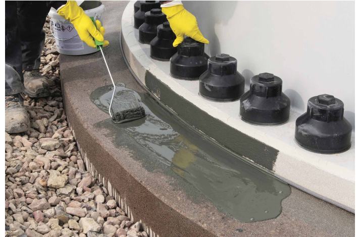
Using a roller to spread the material.
