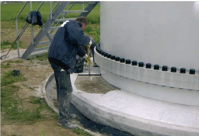
Priming the substrate.
