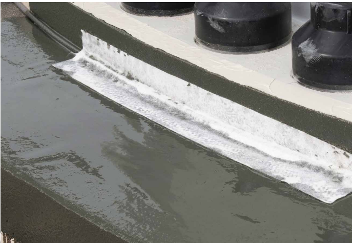
Inserting the fleece on top of the PE Round Cord.
